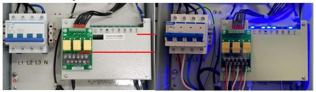
L1, L2, L3 on SEC1000 phases cable must be the same phase cables on inverters L1, L3 and L3. The CTs on A, B, C on the CTs board must be from phase L1, L2, L3 accordingly.
